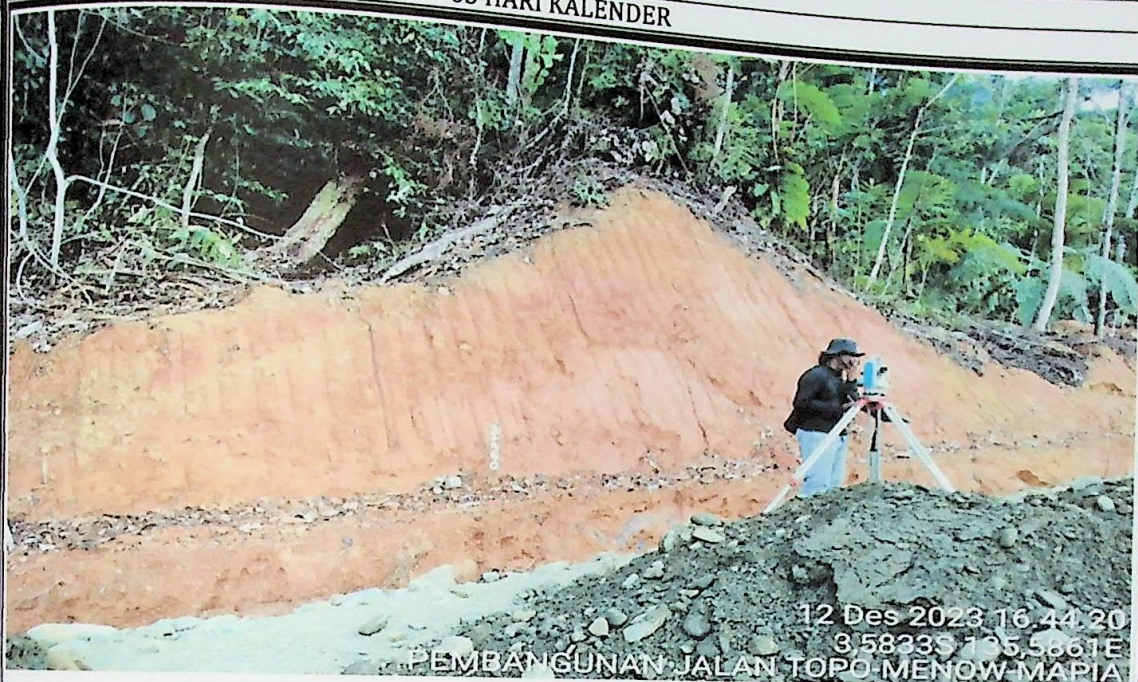
Pekerjaan pengukuran as bult drawing
