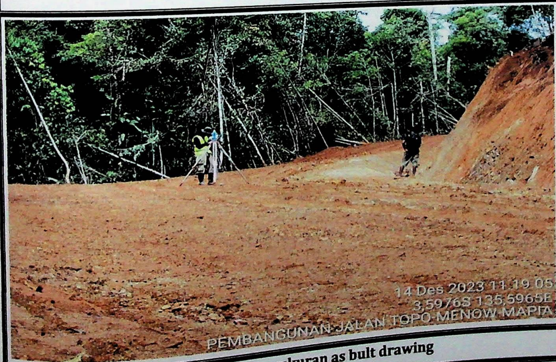
Pekerjaan pengukuran as bult drawing
