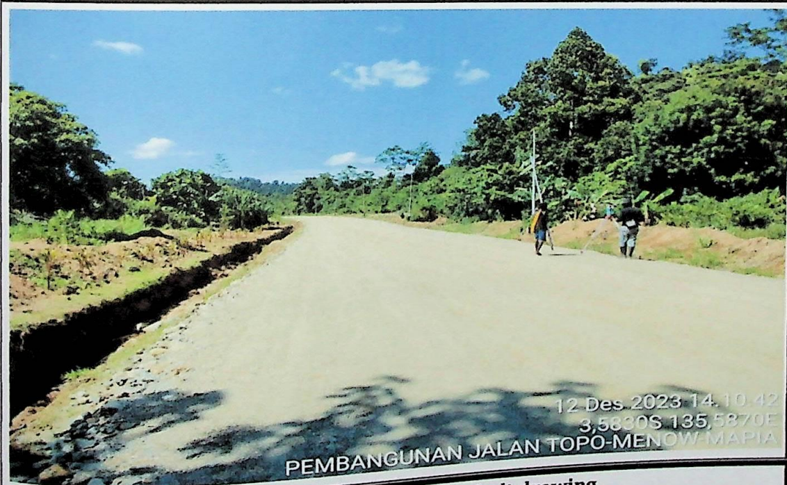
Pekerjaan pengukuran as bult drawing
