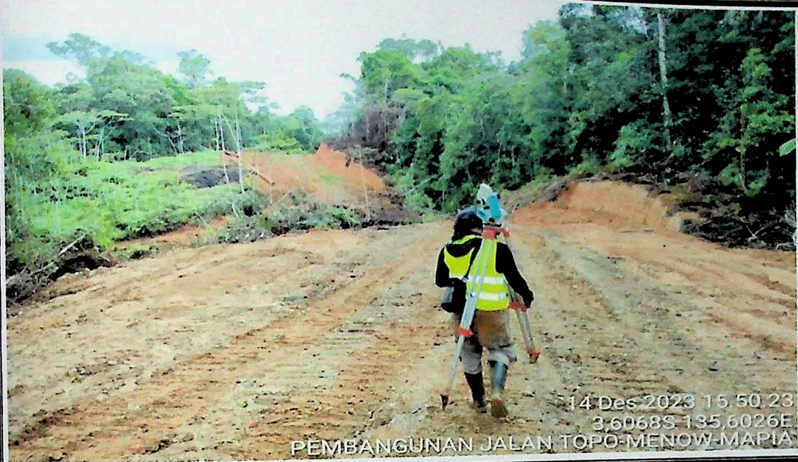
Pekerjaan pengukuran as bult drawing
