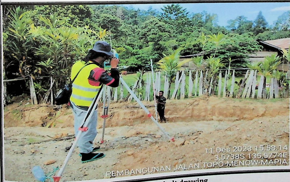
Pekerjaan pengukuran as bult drawing
