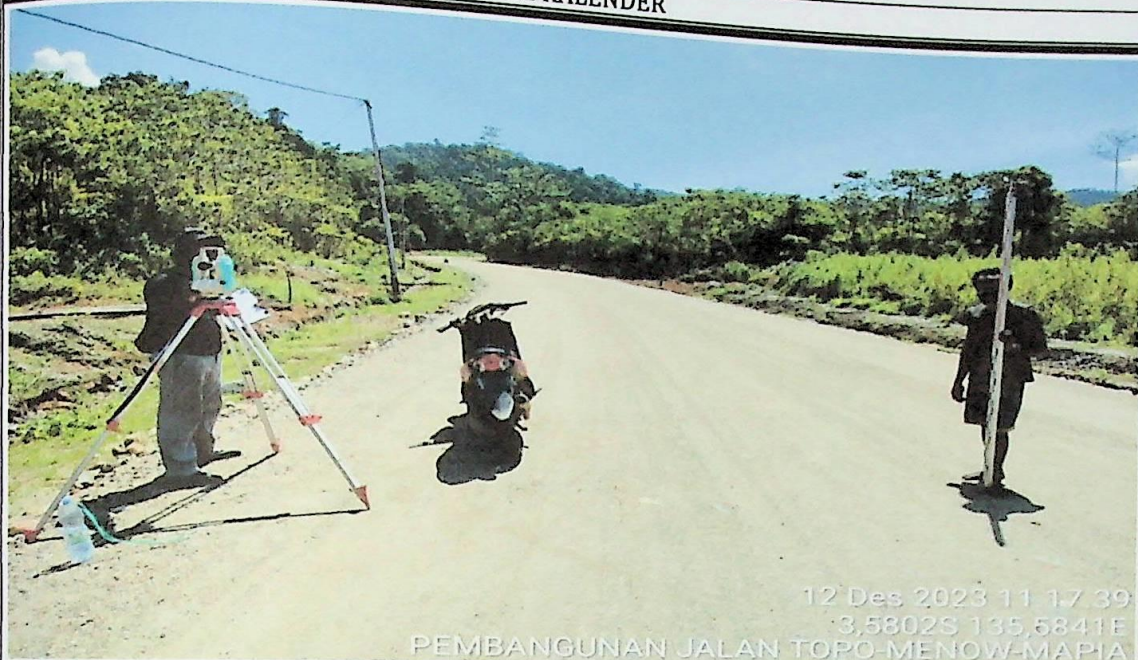
Pekerjaan pengukuran as bult drawing
