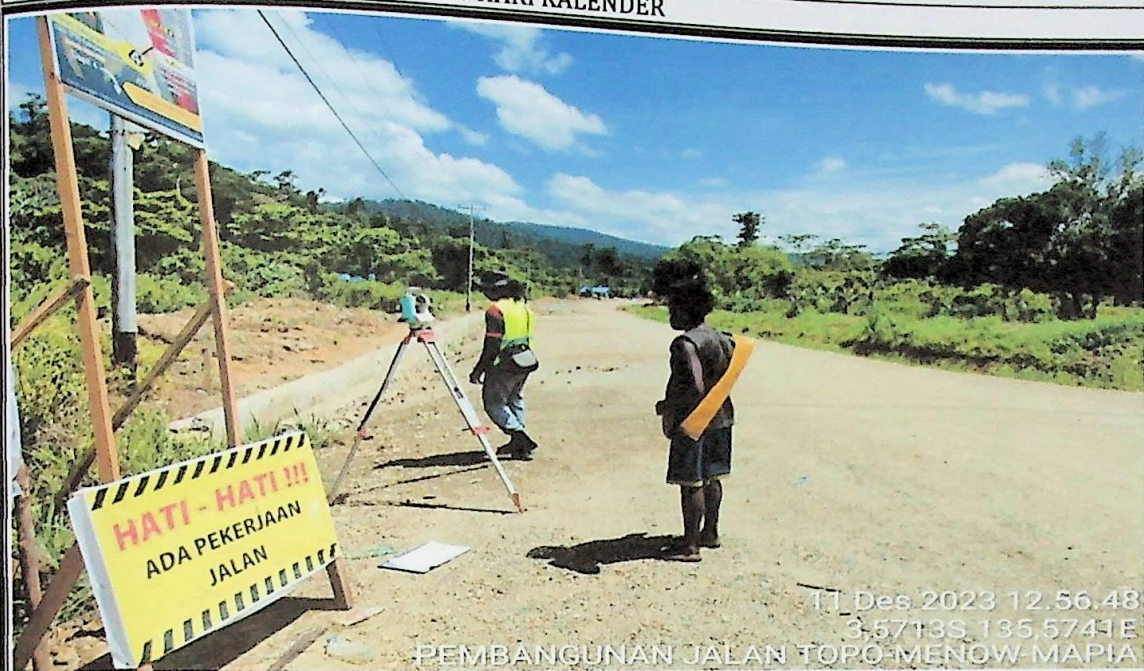
Pekerjaan pengukuran as bult drawing
