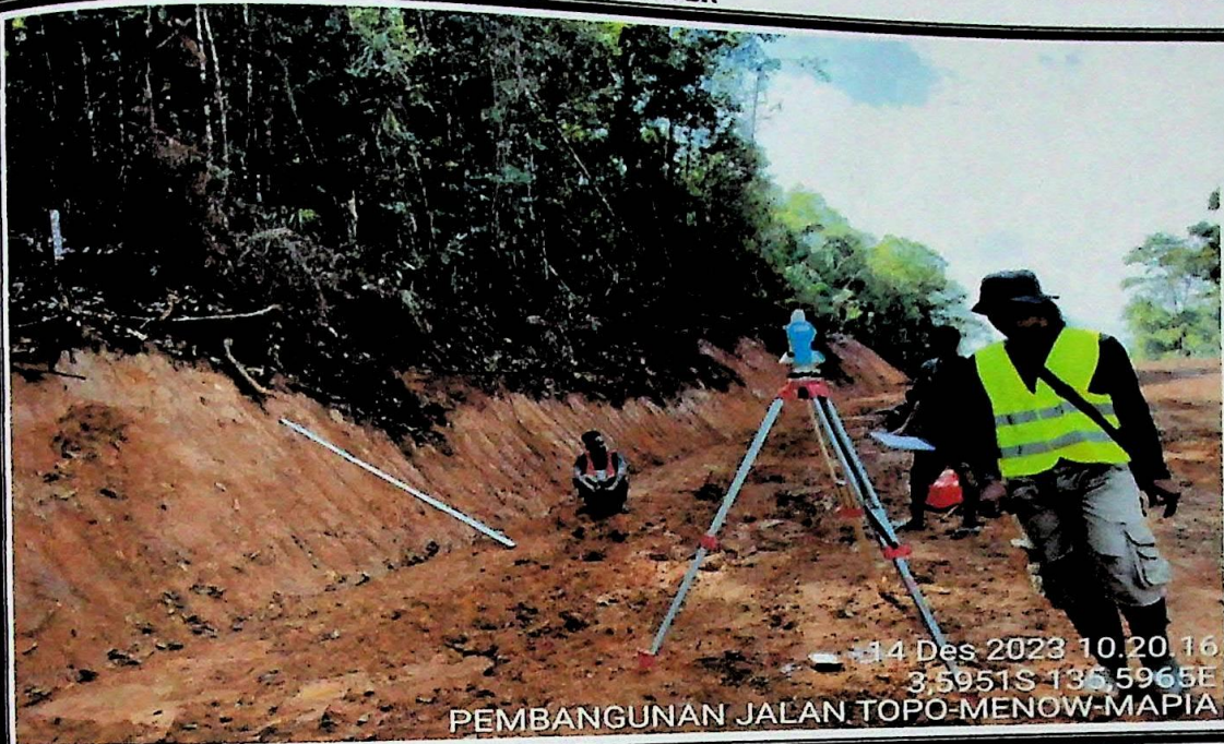
Pekerjaan pengukuran as bult drawing
